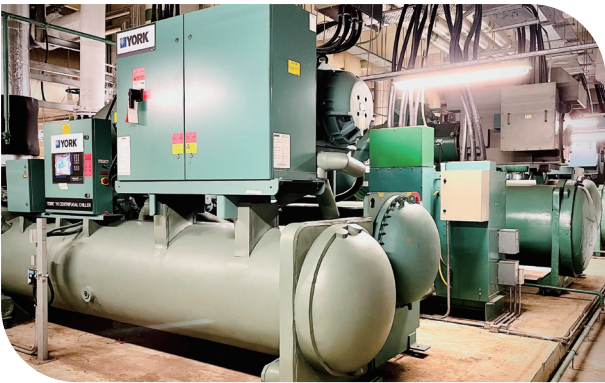
A total of six new heat exchangers and two new chiller units now serve the Cyberport community, saving 200,000kWh and 1,300,000kWh of energy, respectively. 目前共有六台新的热交换器和两台新的冷水机组为数码港社群服务， 分别节约200,000千瓦小时和1,300,000千瓦小时能源。
